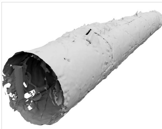
Fig. 4: 3D image of the test section before the emplacement of the HE-E experiment
