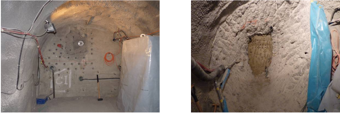
Figure 9: Plug dismantling process (holes around the main one and bentonite reached)
