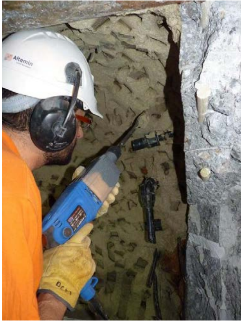
Figure 10: Removal of GBM and bentonite blocks
