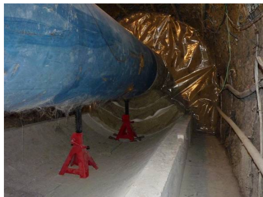
Figure 13: Final metallic beam and sawhorses supporting the canister
