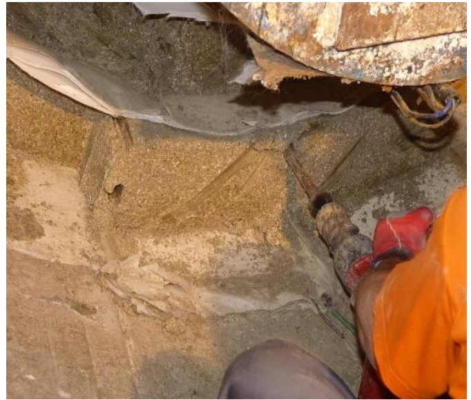
Figure 10: Removal of GBM and bentonite blocks
