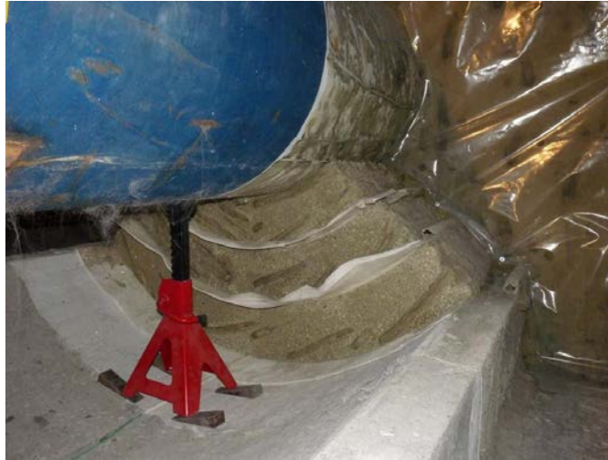
Figure 12: Bentonite (blocks and GBM) and canister left in place for future demonstrator
