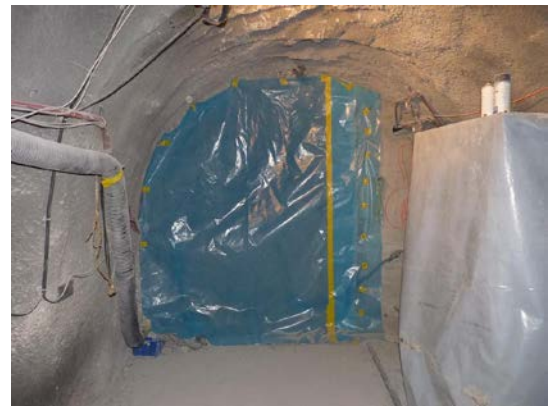
Figure 11: Drying of bentonite (after 5 days) and plastic for protection
