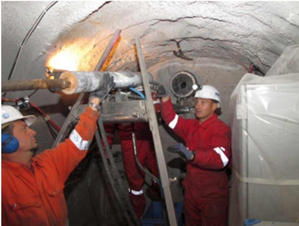
Figure 4: Drilling operation in the EB niche in borehole BEB-PB2
