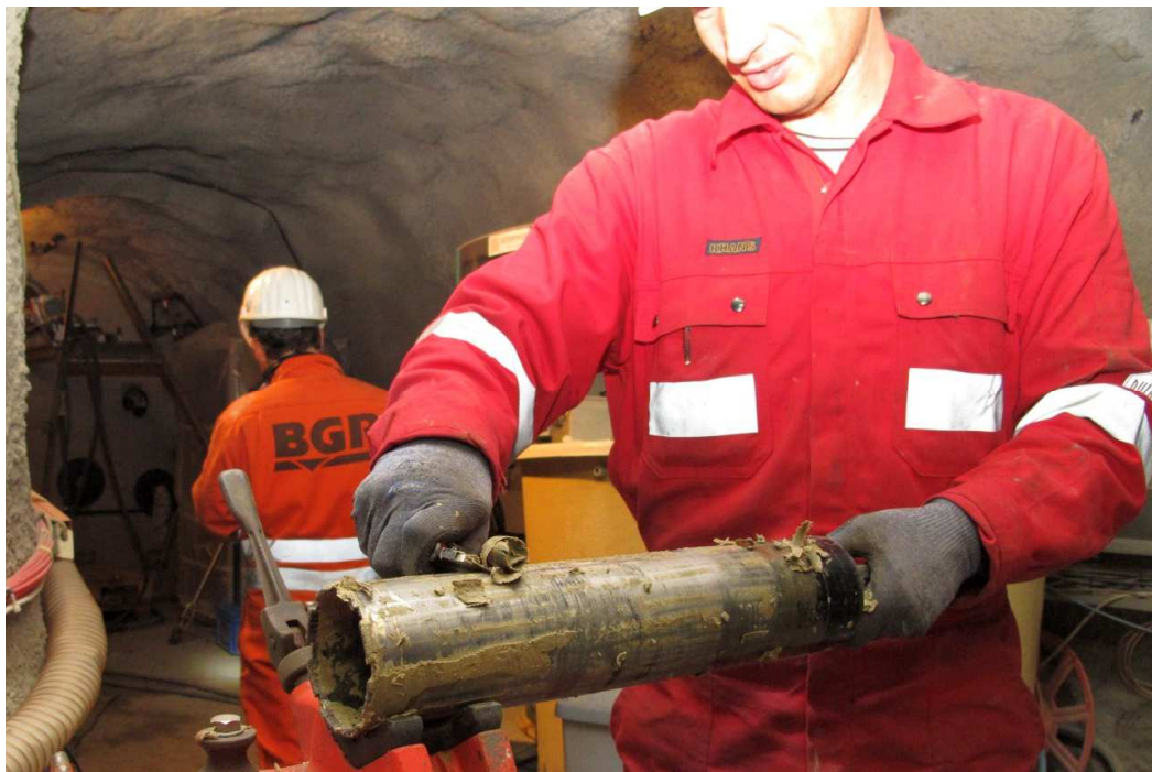
Figure 5: Cleaning of a drilling rod, clotted with bentonite
