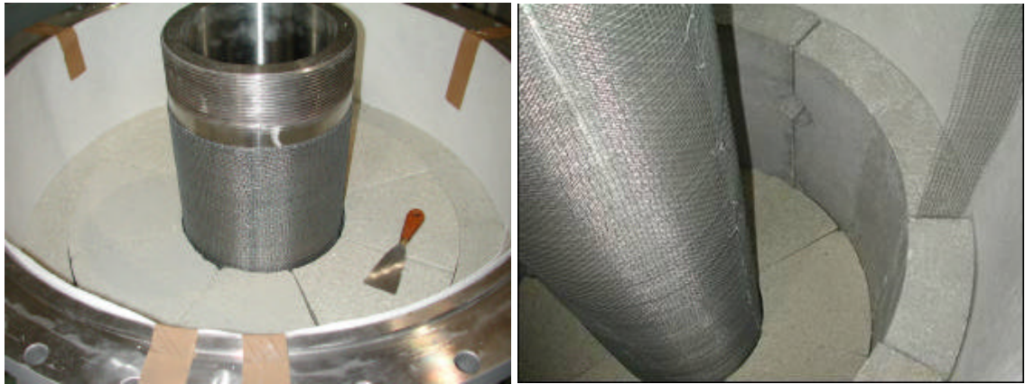
Figure 2-10: Installation of the barrier: clay and concrete/clay tests.
