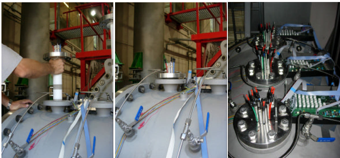
Figure 2-12: Installation of the instrumentation rods and connection to DAS.
