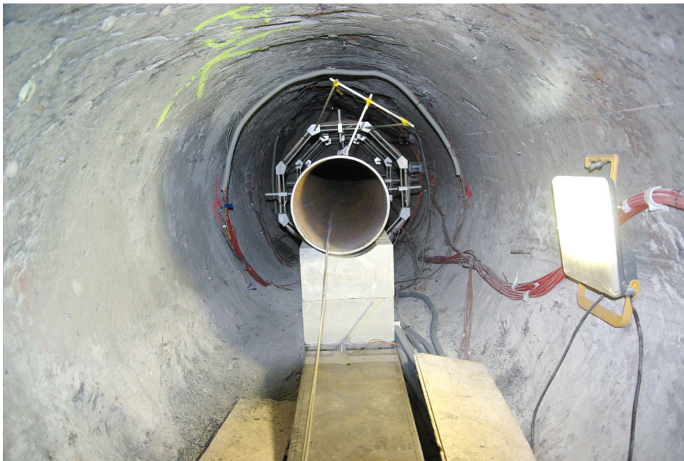
Fig. 6.21: Liner, bentonite blocks, and instrumentation in the sand/bentonite section.
