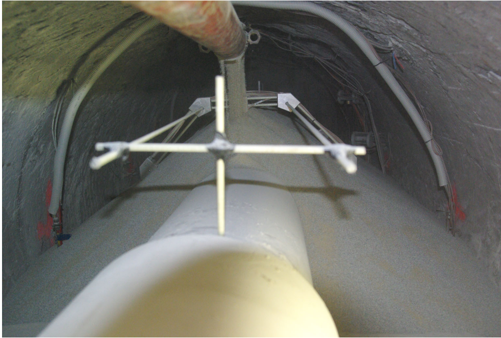
Fig. 6.24: Sand/bentonite emplacement.
