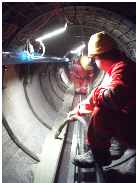
Fig. 2.14: Concreting of railway system (picture from Implenia).
