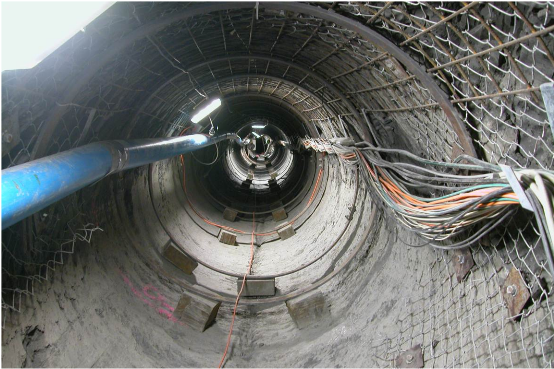
Fig. 2.9: Microtunnel cleanup phase before initiating activities for the HE-E experiment showing the presence of the steel rings hindering the emplacement of the railway system (font from Solexperts).
