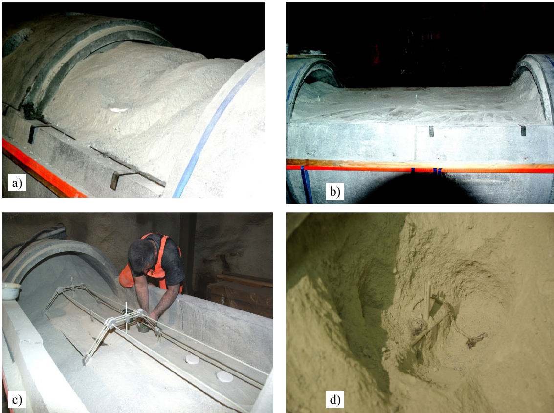
Fig.3.11: a) – b) Test sections after dismantling the roof of the concrete tube; c) bentonite sampling with cutter cylinders; d) damaged sensor carrier element
