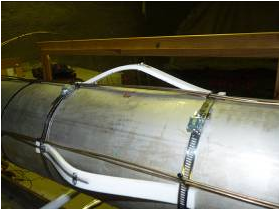
Photographs 4.3.7: Detail of the positioning Teflon pieces
