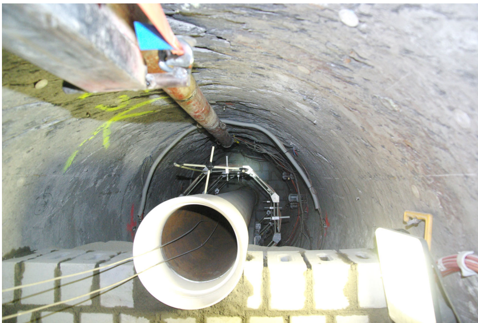
Fig. 6.23: Start of sand/bentonite emplacement.
