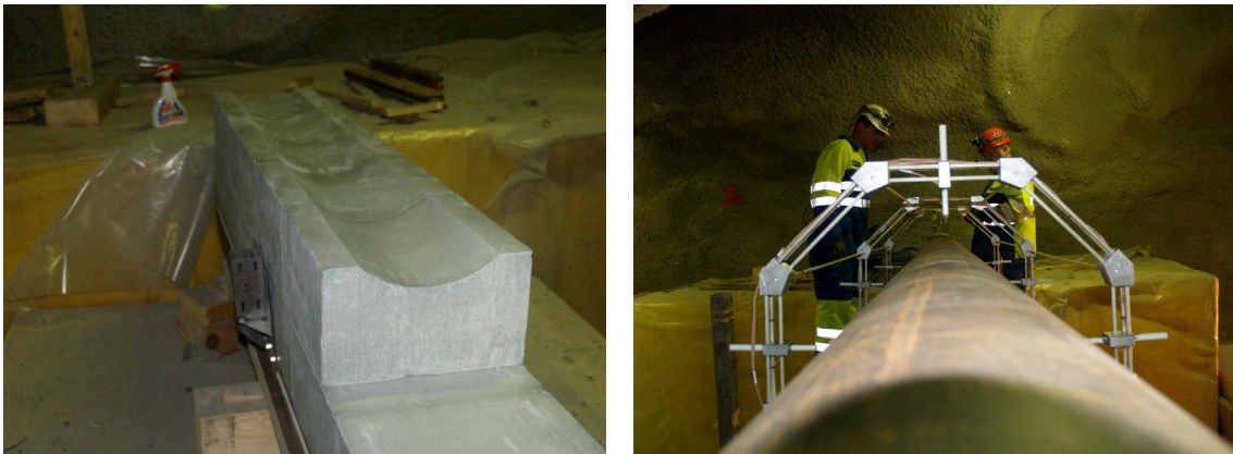
Fig. 6.10: Construction of the instrumentation modules on the platform.
