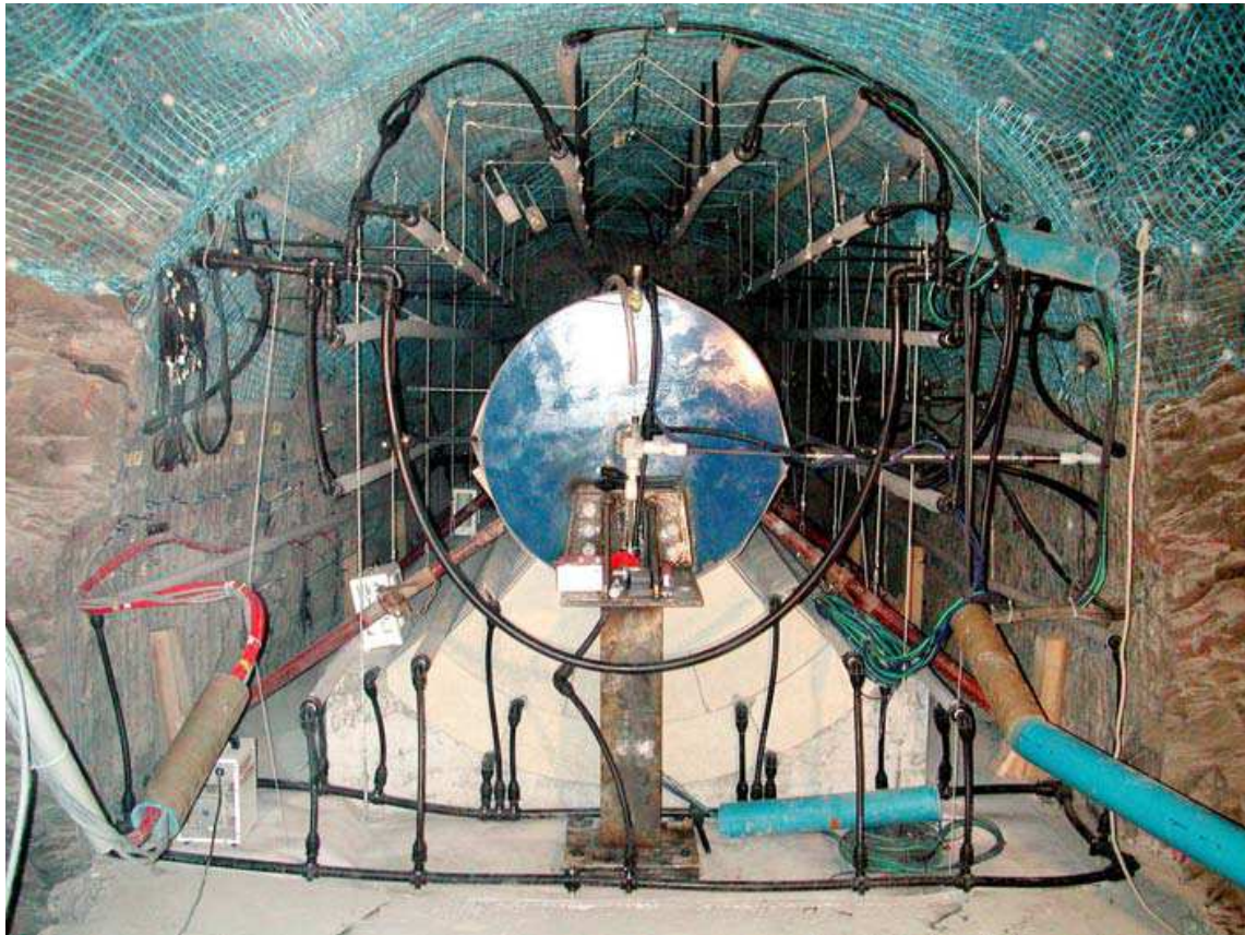
Figure 2: Appearance of the concrete and bentonite blocks bed, dummy canister and hydration system before the installation of the GBM (ENRESA 2005)
