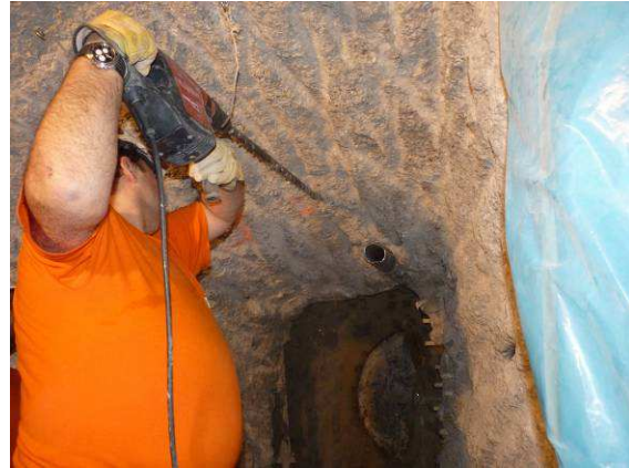
Drilling boreholes for the expansive cement (II)
