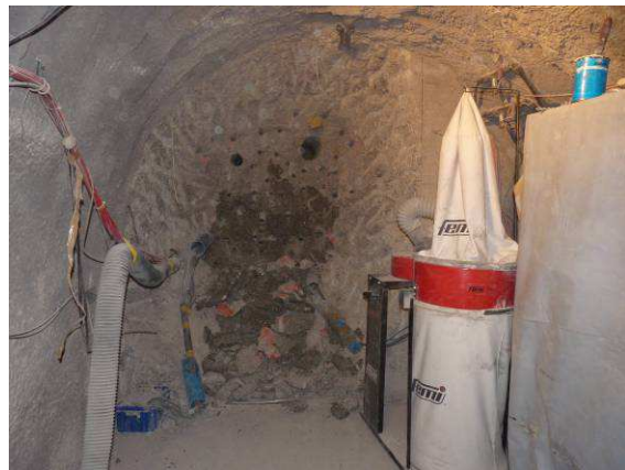
Retaining wall dismantling
