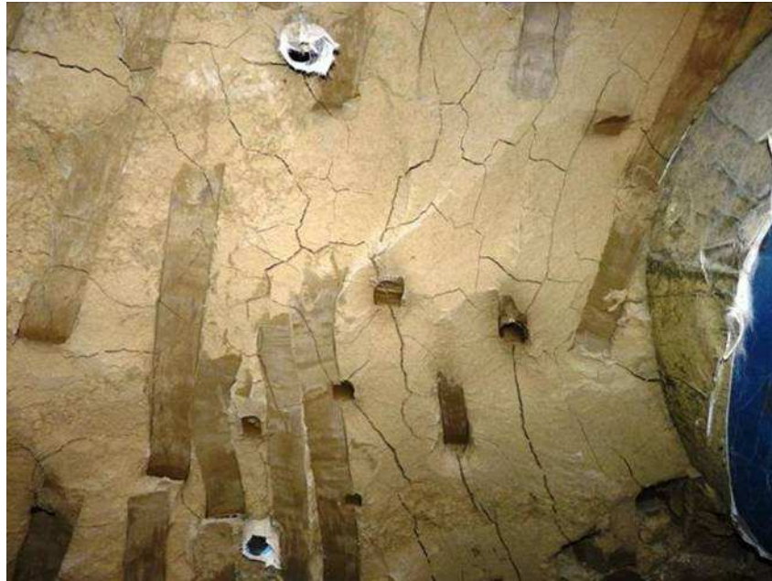
Figure 21: Bentonite front dryness after 5 days exposed
