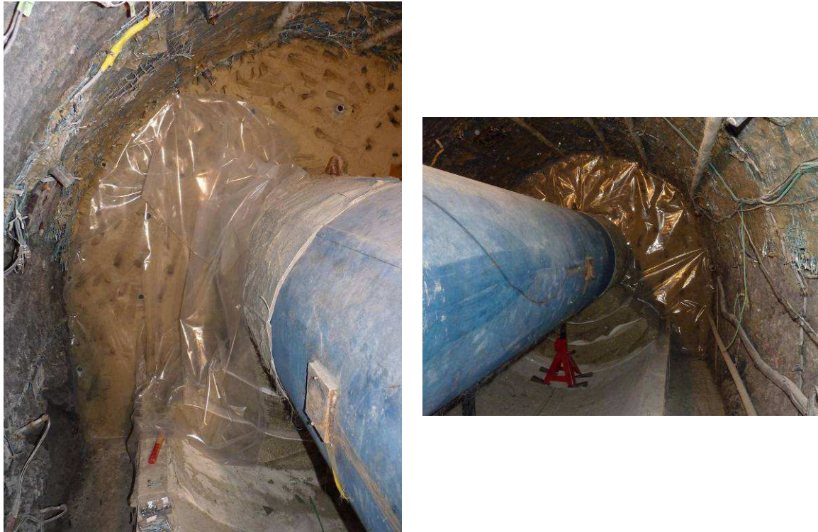
Figure 26: Front of the remaining bentonite covered with plastic
