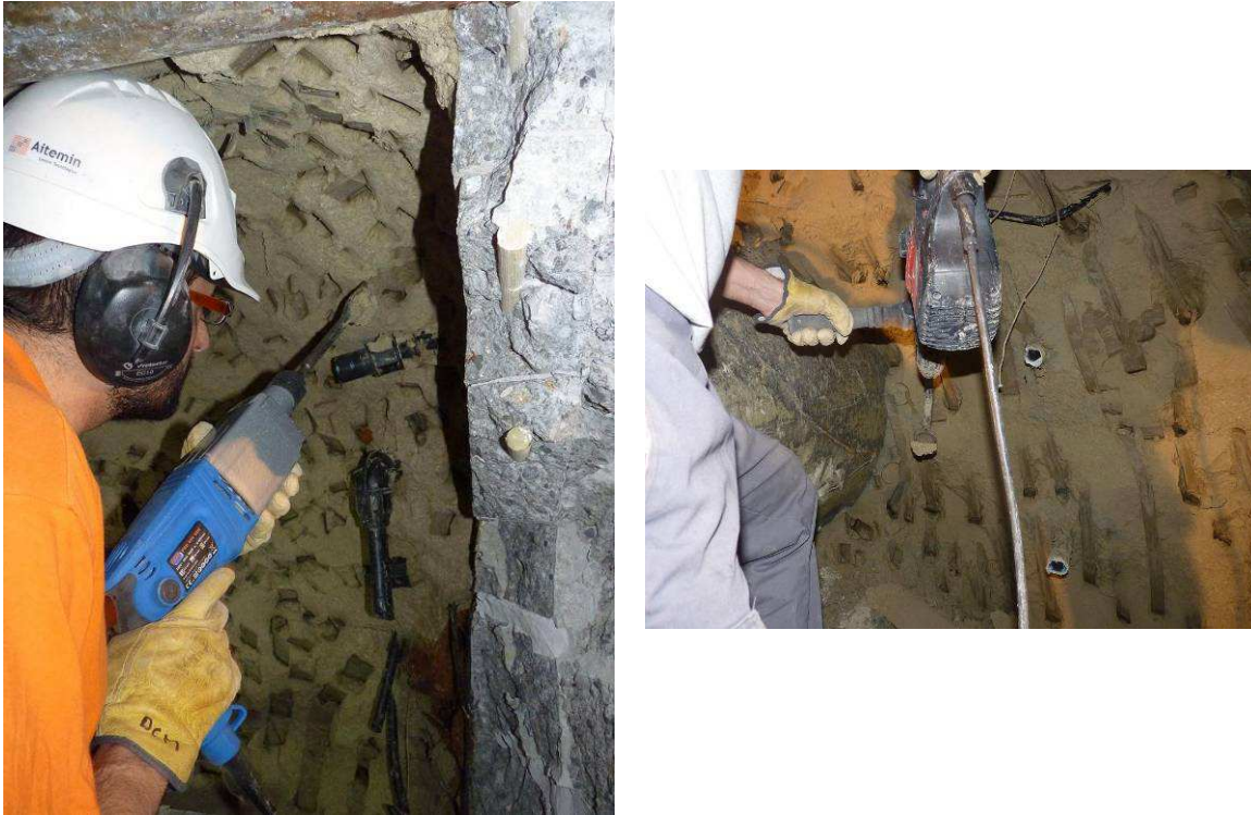
Figure 19: Tools used for bentonite removal
