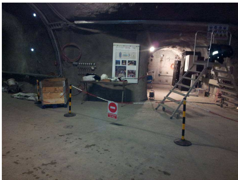
Figure 5: Installation of safety signs
