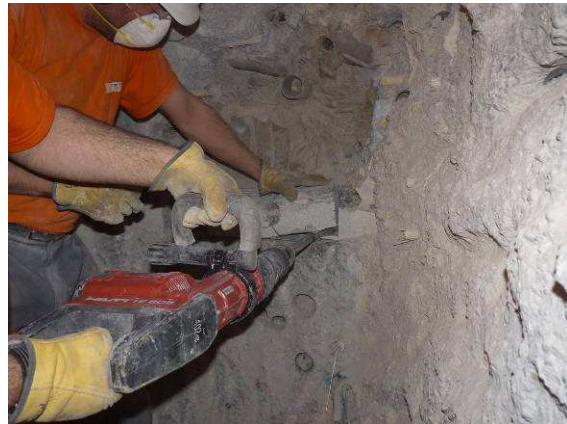
Sampling the concrete/bentonite interface of the retaining wall as a block
