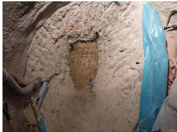
Bentonite in contact with the retaining wall
