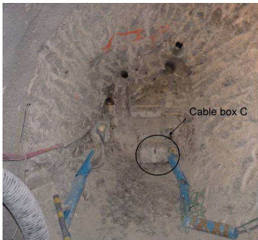
Reaching the cable box C
