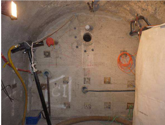
Boreholes around the 200 mm diameter one
