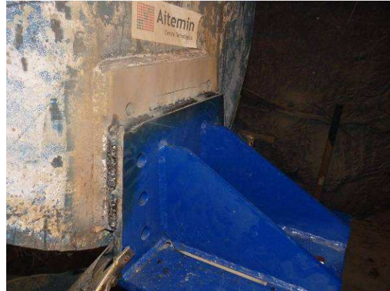
Metallic beam already welded to the canister front
