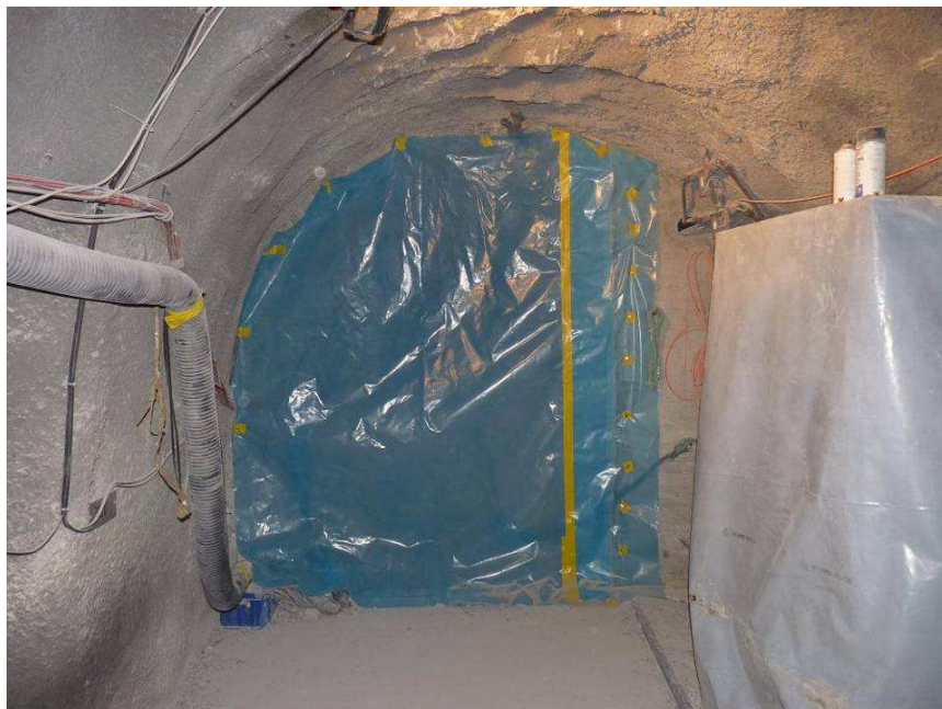
Figure 22: Plastic cover to avoid bentonite drying
