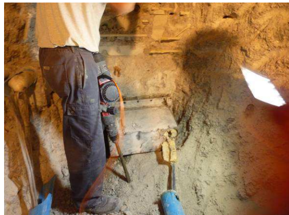
Cable box C dismantling (I)
