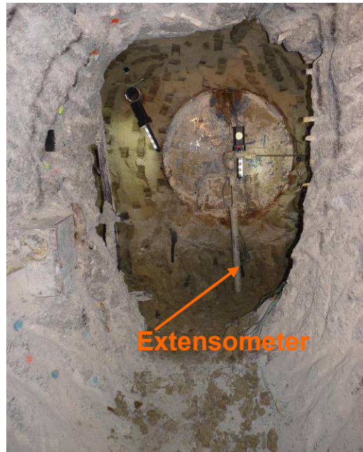
Front face of the canister and vertical extensometer uncovered. Section A1
