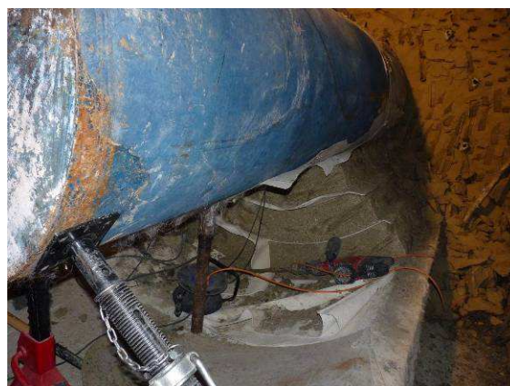
Temporary support of the canister
