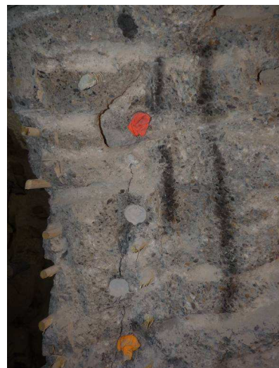
Insertion of solid expansive cement in lateral and top boreholes
