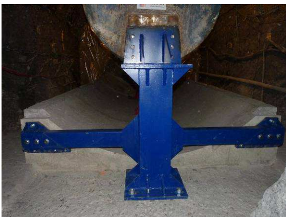
Front view of the metallic beam
