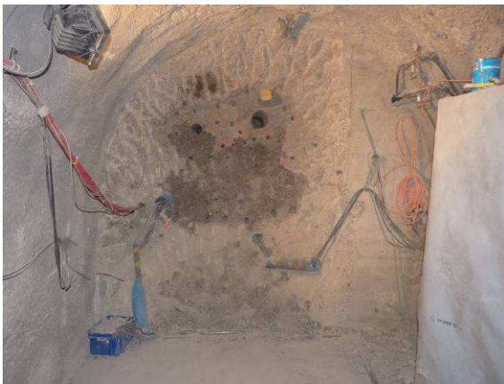
Retaining wall reached
