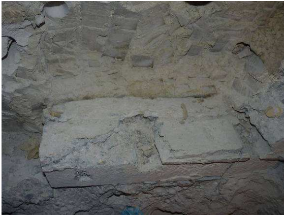
Retaining wall. Concrete/bentonite interface
