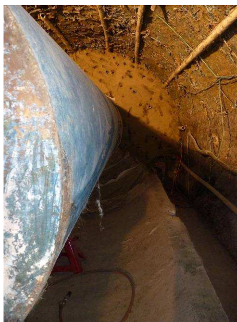
End of the bentonite removal. Z=695 for the GBM
