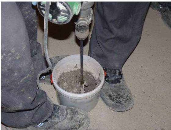
Preparation of the liquid expansive cement
