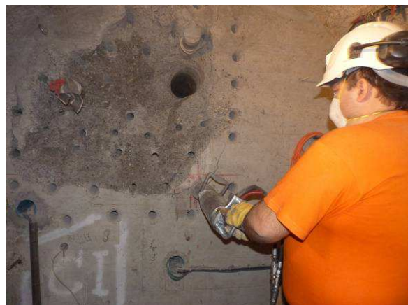
Use of the Darda to break the concrete
