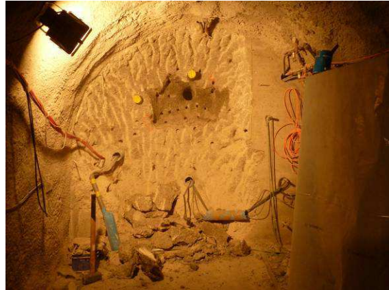
Result of the use of the backhoe
