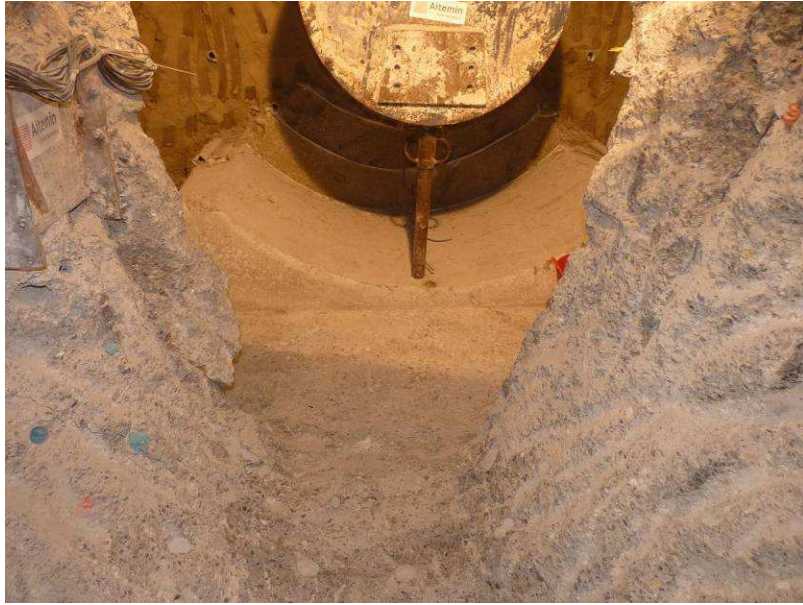
Figure 27: Metallic extensible support for canister
