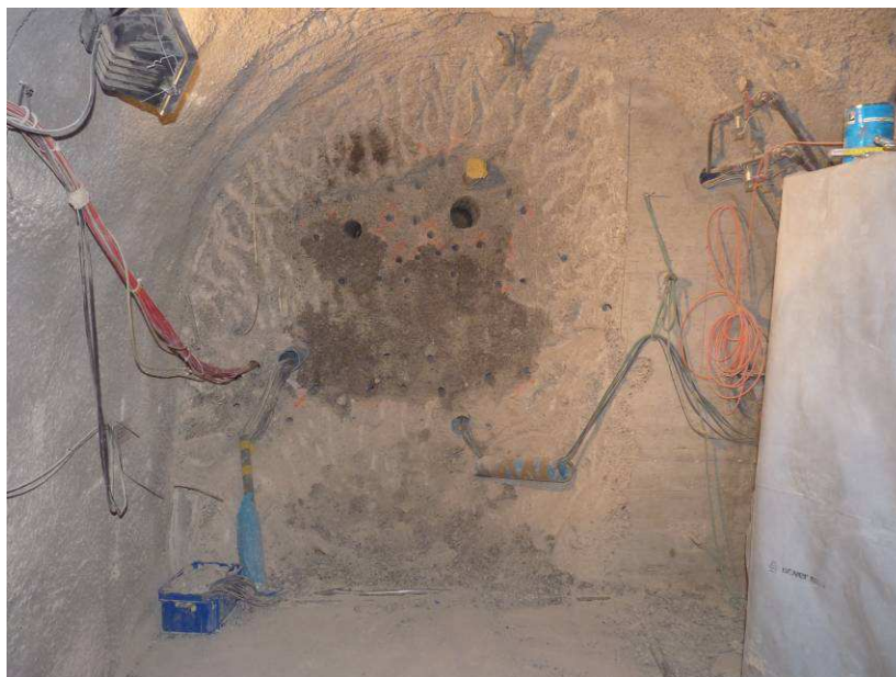
Figure 47: Wet concrete. Plug
