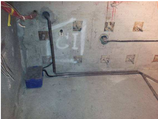
Figure 3: Protection of seismic cables
