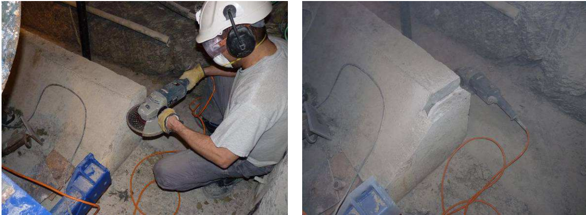
Figure 35: Concrete bed sampling
