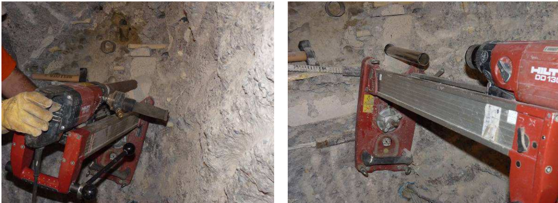
Use of the rotating coring equipment for the concrete part
