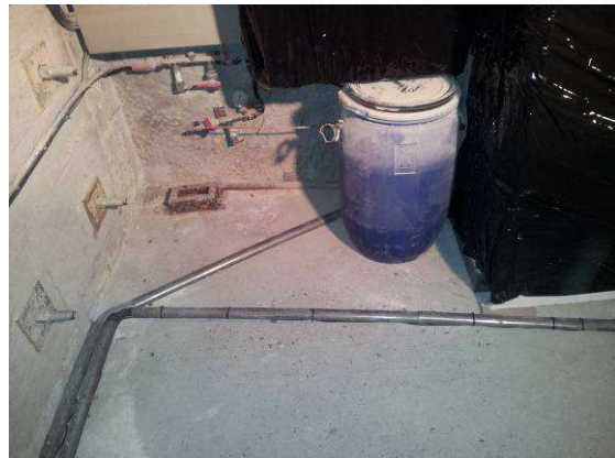
Figure 3: Protection of seismic cables
