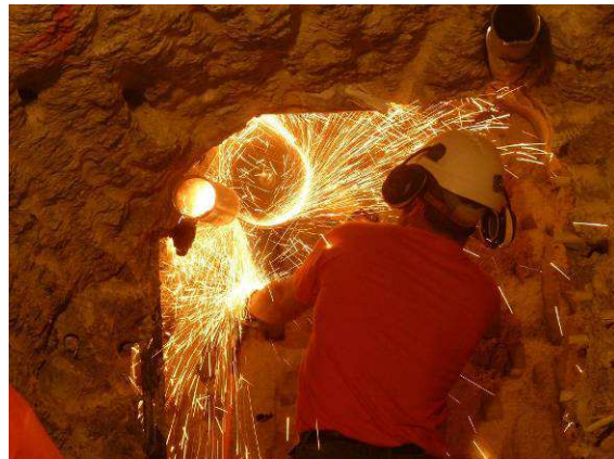
Cutting of the steel pipes located along the experiment
