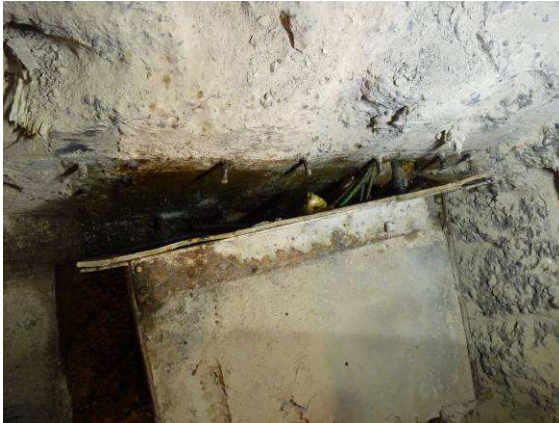
Cable box C dismantling (II)
