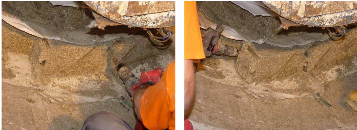
Figure 20: Tools for bentonite blocks removal
