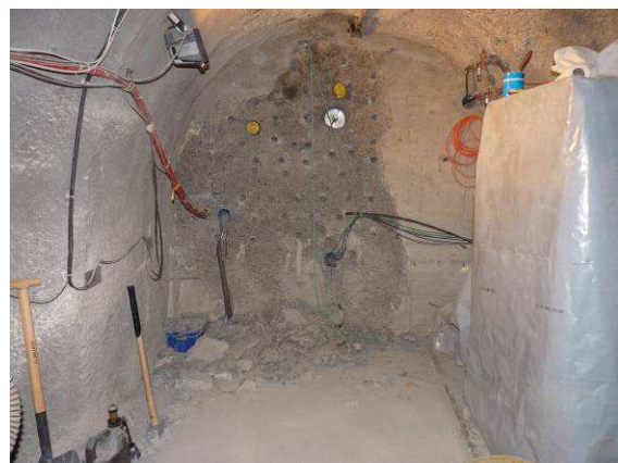
Progress in breaking the concrete of the plug
