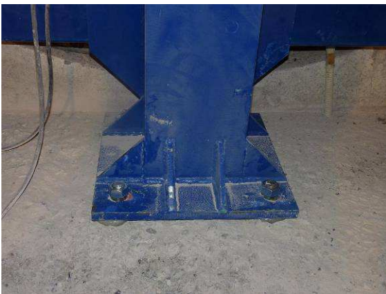
Attachment of the bottom part of the beam to the floor
