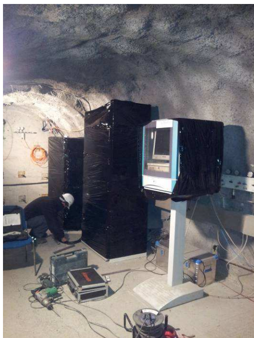
Figure 4: Protection of the cabinets
