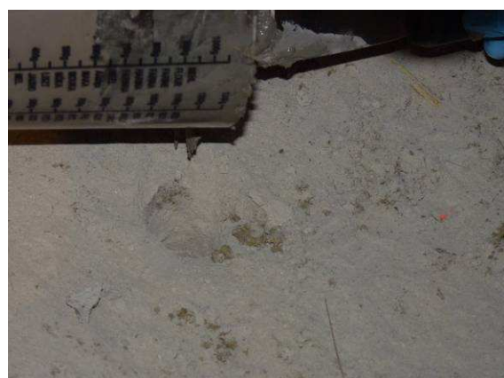
Pouring of liquid expansive cement in the floor boreholes
