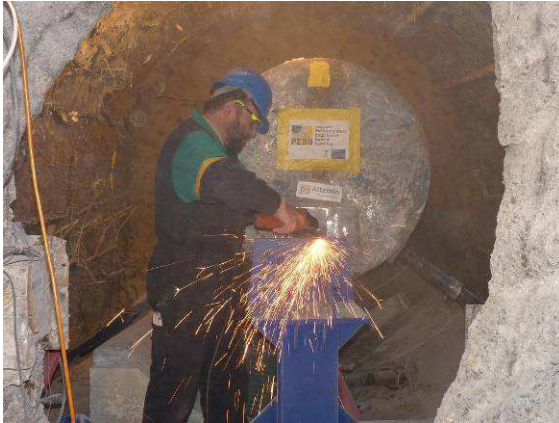
Welding of the beam to the front face of the canister
