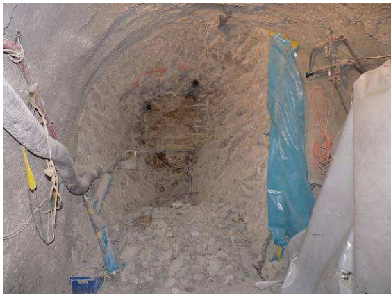
Reaching retaining wall and bentonite
