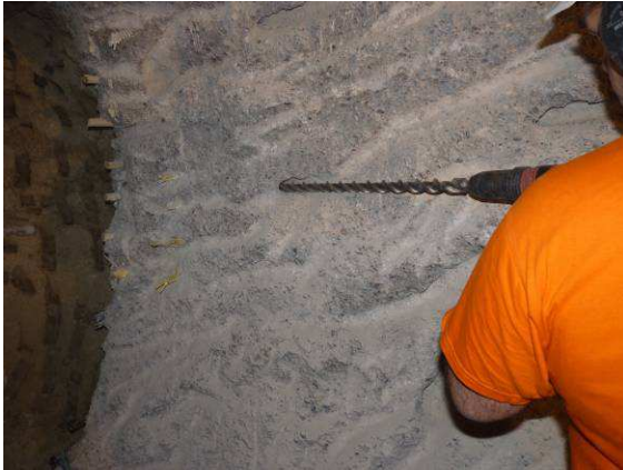
Drilling boreholes for the expansive cement (I)
