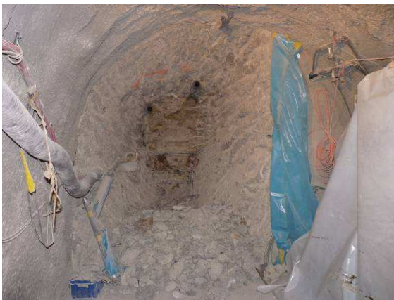
Retaining wall dismantling
